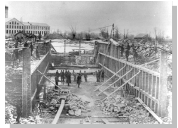
Construction of the Fox River Locks, 1840s
